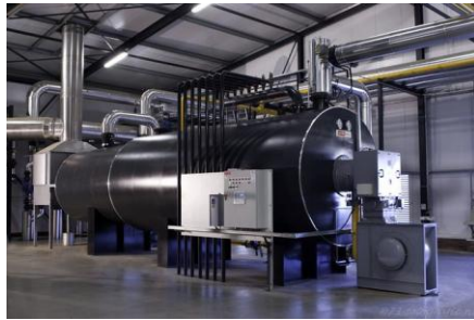
Hydrogen boilers
